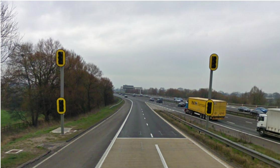
Figure 2.20: Example of an on-ramp controlled by a ramp metering system in an English motorway. Adapted from TeleAtlas (2013).
