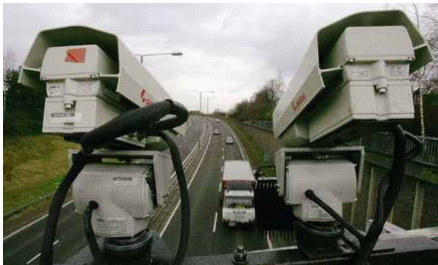
Figure 2-3 Photograph of CCTV Camera Used to Monitor Traffic Flow (Guardian 2011)
